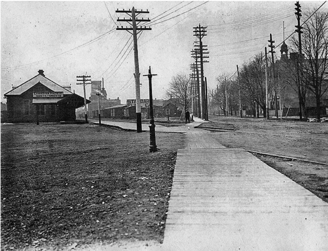
View along Cottingham St. west from Yonge circa 1900. Note the CPR station on the left behind which a grain elevator can be seen, presumably on the property where the tennis club now stands. Notice the bell tower of Cottingham Public School on the right. [Photo courtesy of City of Toronto Archives.]
